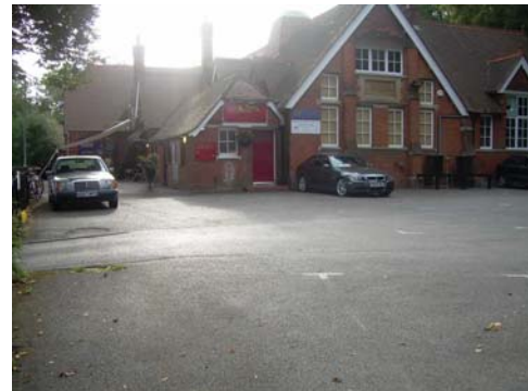
Photo 2.4 Main Centre building & car park
